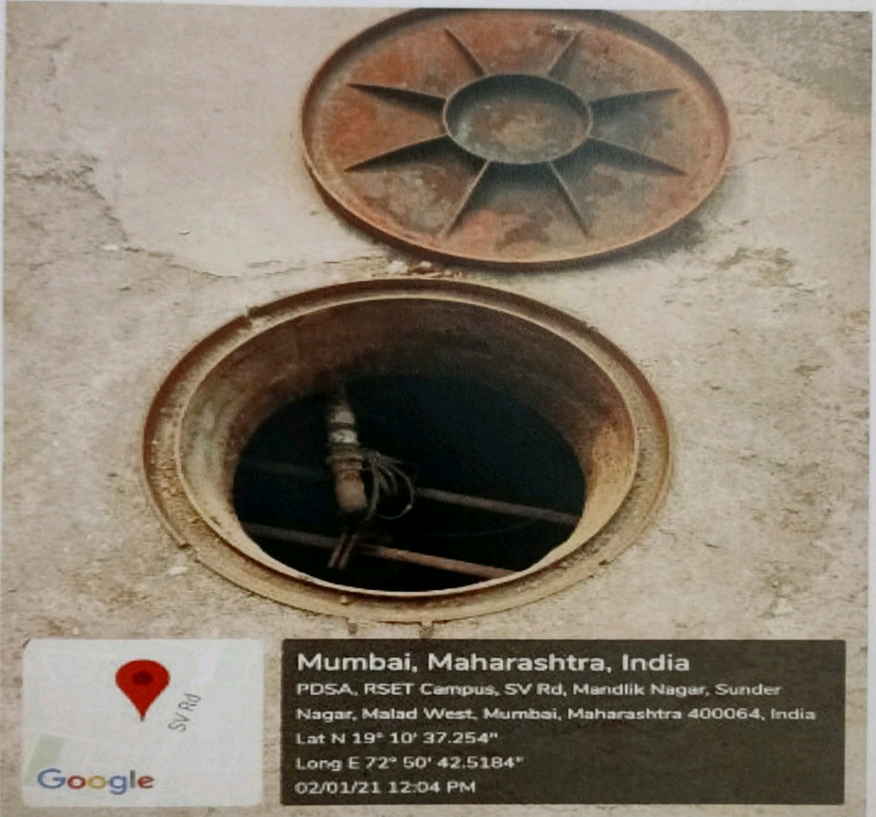
Bore well picture 2
