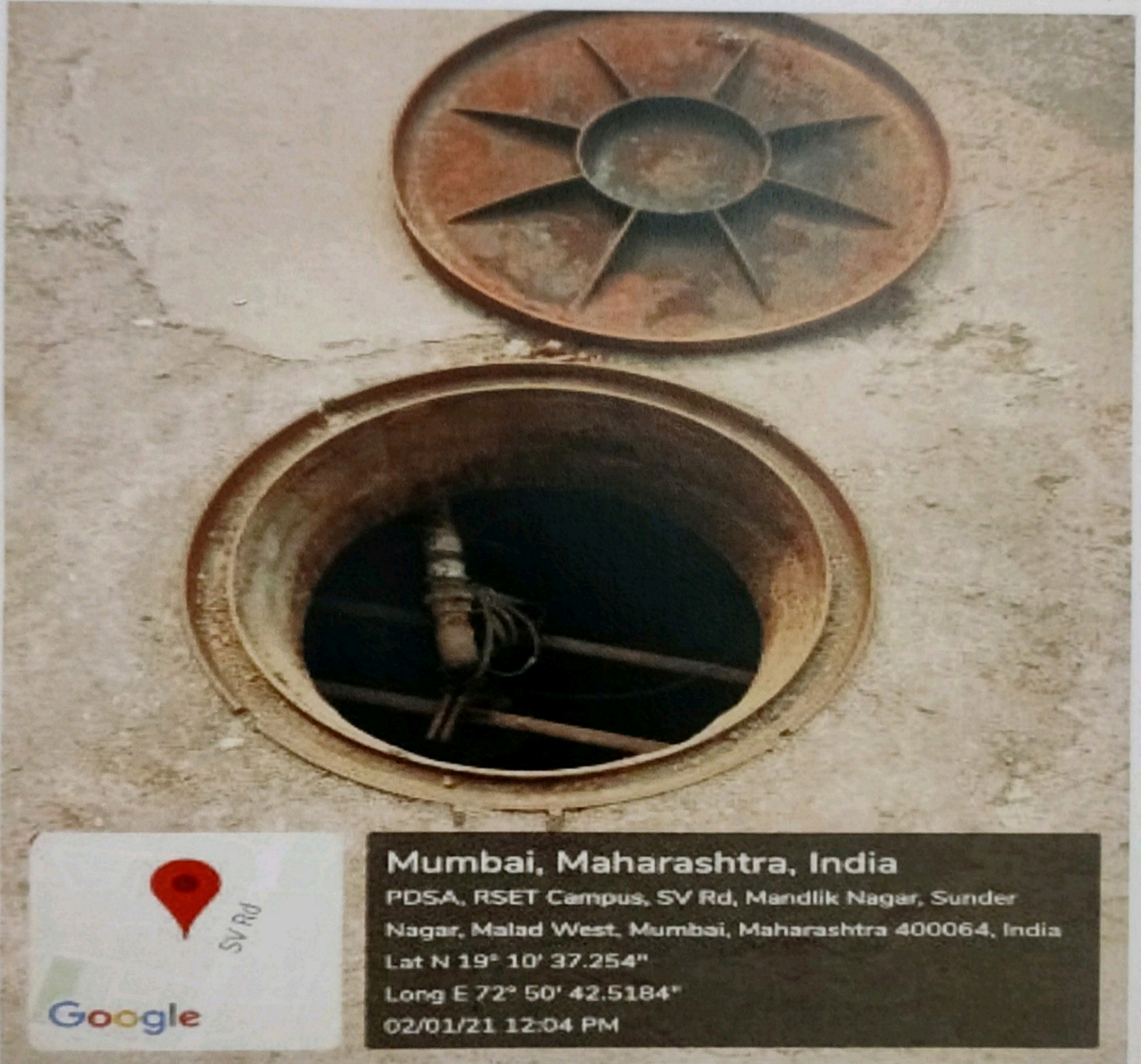
Bore well picture 2
