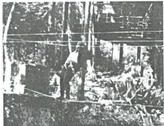
Parallel Bridge Crossing
